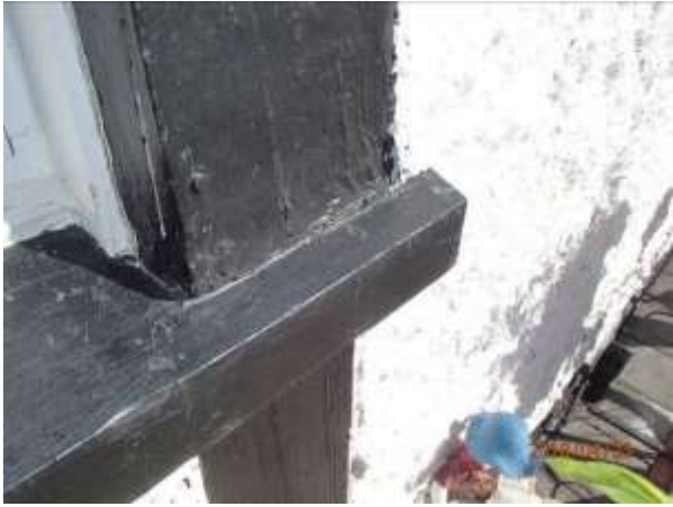
The bottoms of the facings are all starting to fail.
