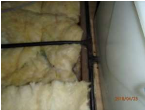
Steel conduits appear to still be in use; images show the conduit in the roof and the light below
