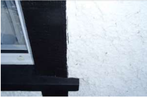
All of the opened junctions need to be sealed.
