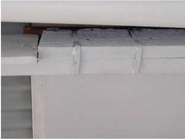
The top end of the carport rafters are not that well fixed.
