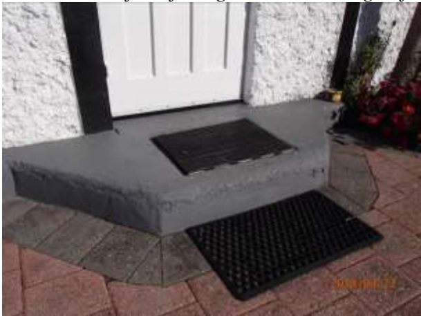
This step is very close to floor level
