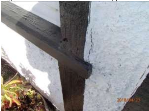
This facing should be replaced
