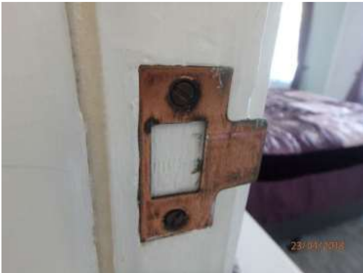
Has not been housed out for the latch
