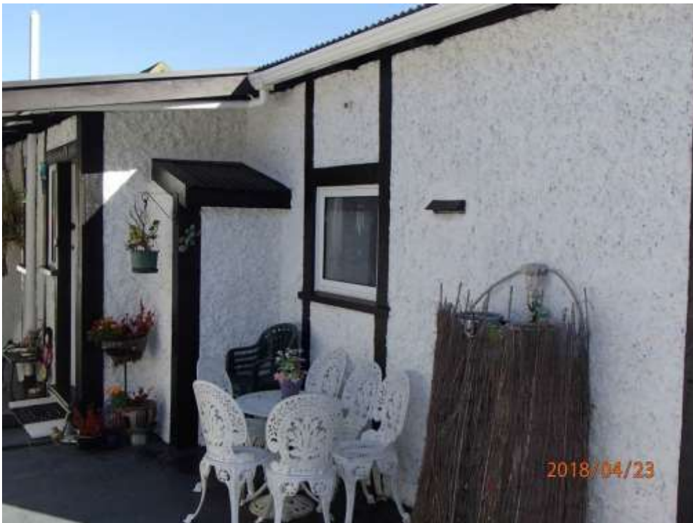
On this side are the carport and storage lockers along the fence. There is a cut off drain in the carport to control surface water which is discharged to a sump. Two 45 Kg gas bottles are hidden behind some brush hedging against the house.
