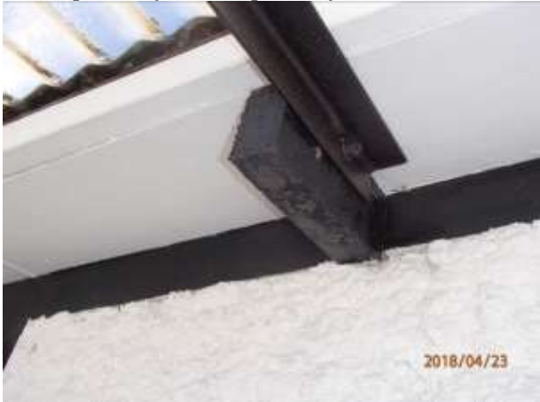
Just one bolt to an undersized steel angle. The outer end is better supported
