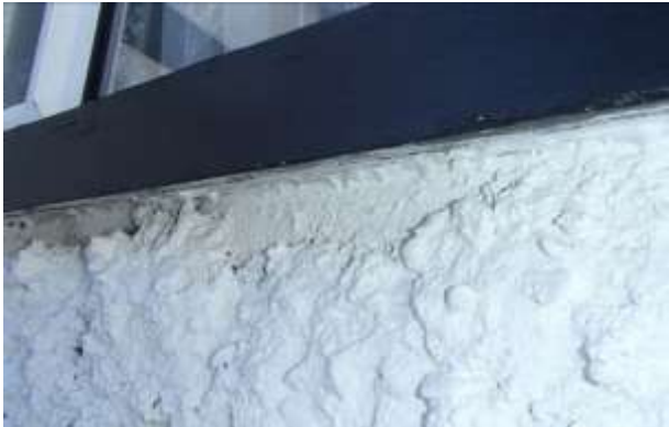
Difficult to tell what the plaster is applied over but it does not look that well done
