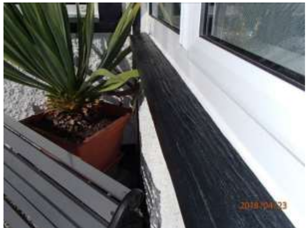
window sill with blistering paint needs some work
