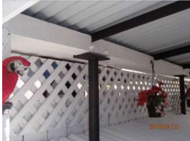
Just one bolt to an undersized steel angle. The outer end is better supported
